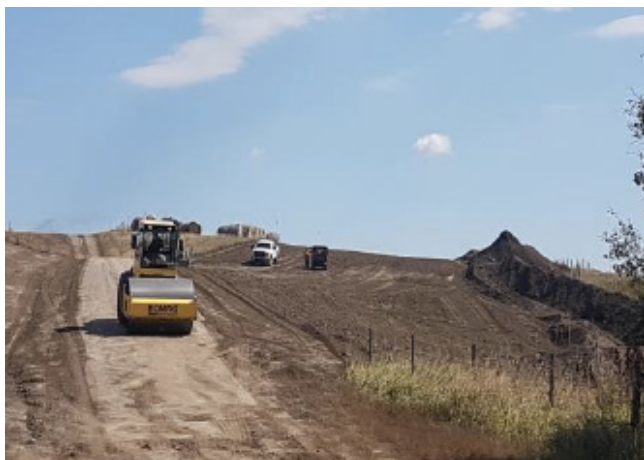
Roller packing soil on ROW– SF 22 – Aug 31, 2018
