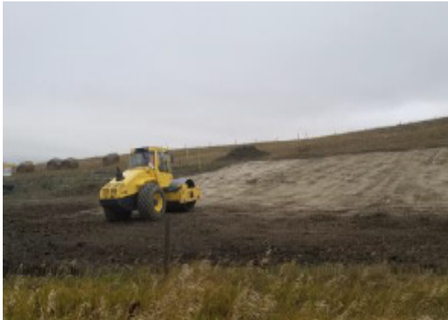
Drum roller packing – SF 9, Aug 27, 2018
